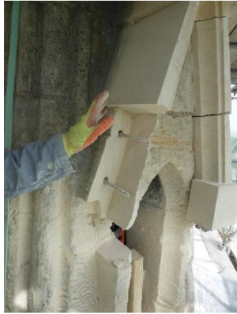
A stonemason holds a corroded iron clamp – the cause of the cracked stones
