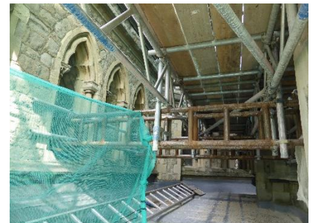
Scaffolding behind the netting in July 2016
