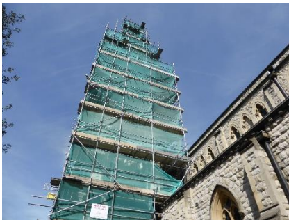
Spire is fully clad in scaffolding and netting in May 2016
