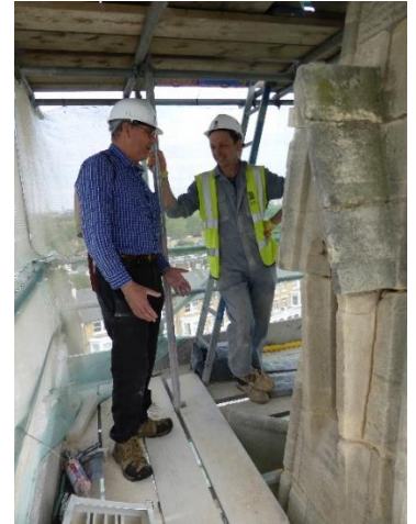
A stonemason holds a corroded iron clamp – the cause of the cracked stones
