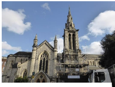
The HLF construction board is mounted 11 February 2016
