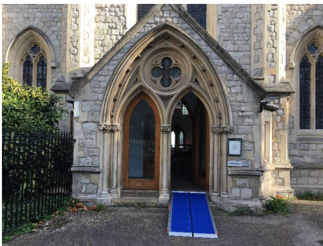
New wheelchair ramp at entrance to Highbury Heritage visitor centre
