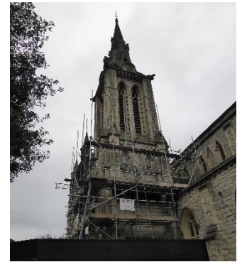
Scaffolding climbs higher 19 February 2016
