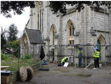
Scaffolding has arrived 10 February 2016
